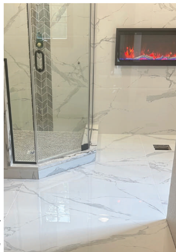
Photo 1: A custom installed shower by Becwar Tile & Marble.
